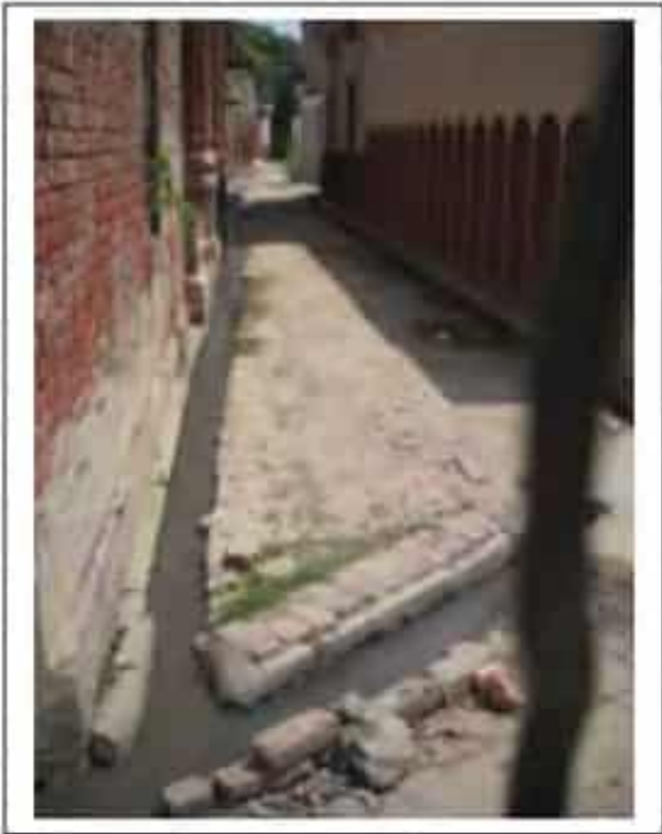
Street before intervention
