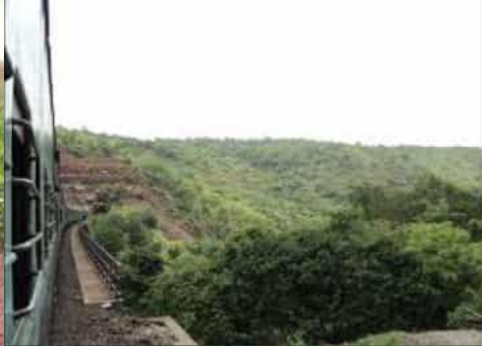
Vetiver embankments on the Bombay-Goa route
